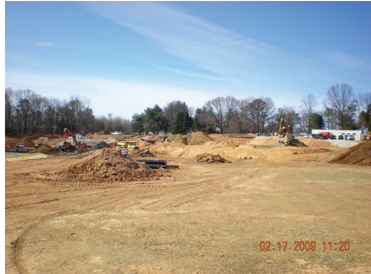
Figure 11 - Site Soil Picture
