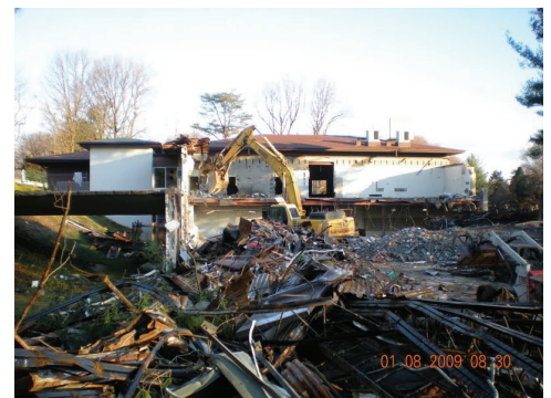
Figure 4 - Demolition of Existing Building
