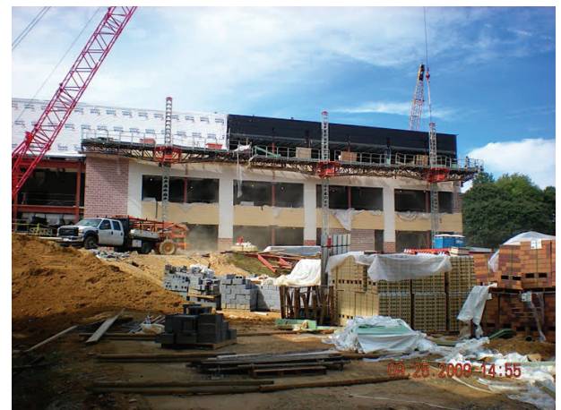
Figure 8 - Masonry Staging Area & Elevation
